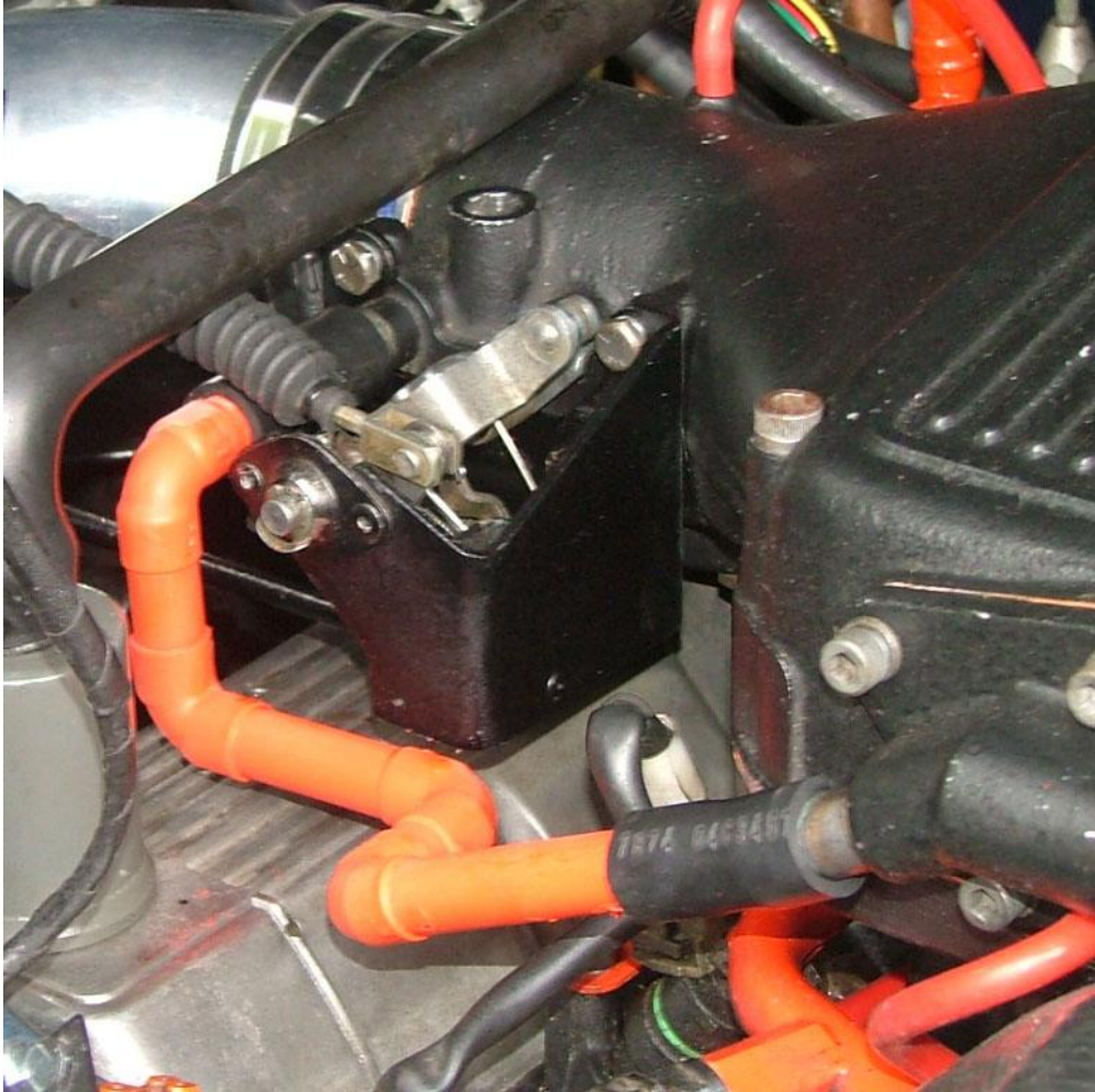
Figure 51 – Idle air supply pipe (red) – finalised
