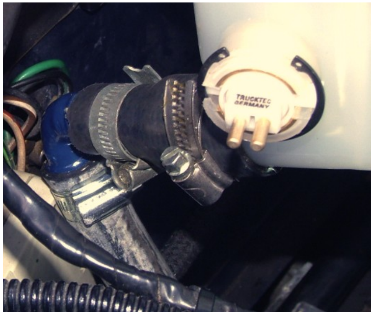
Figure 17 – Expansion tank main feed and copper union
